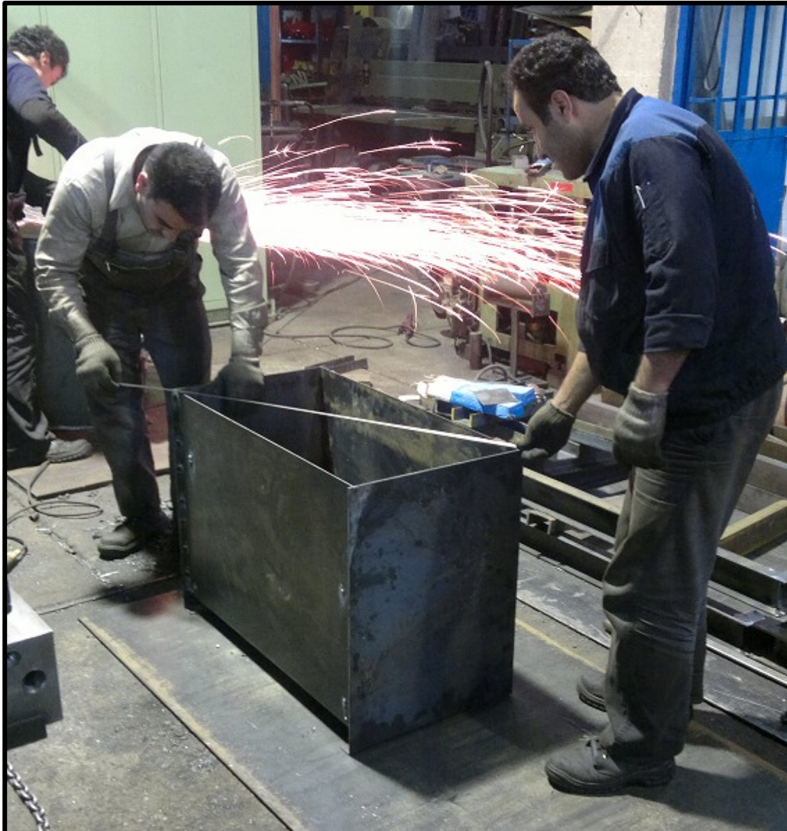
Fig 1 – 3 sets hydraulic tanks have been assembled and are ready for final welding. With respect to customer inquiry these tanks should have 200 Lit volume using 3mm thickness bended carbon steel plates
